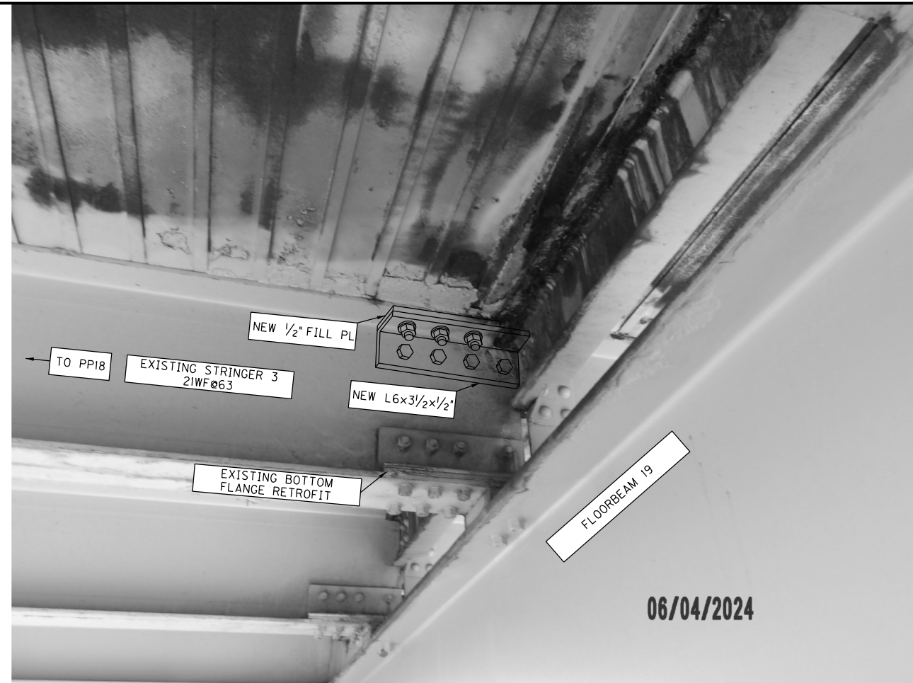
LOOKING SOUTHEAST AT THE NORTH FACE OF FLOORBEAM 19
