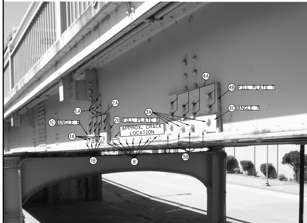
OUTBOARD FACE OF GIRDER 1, SPAN 35, AT FLOORBEAMS 7&8 LOOKING SOUTHWEST
