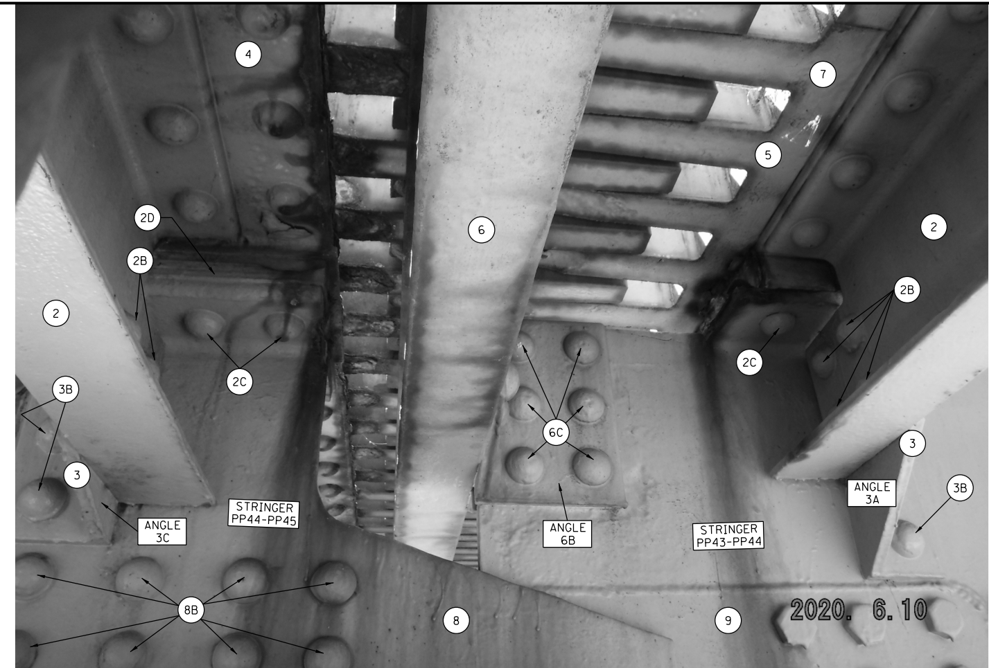
VIEW LOOKING WEST FROM THE CENTERLINE OF PP44
